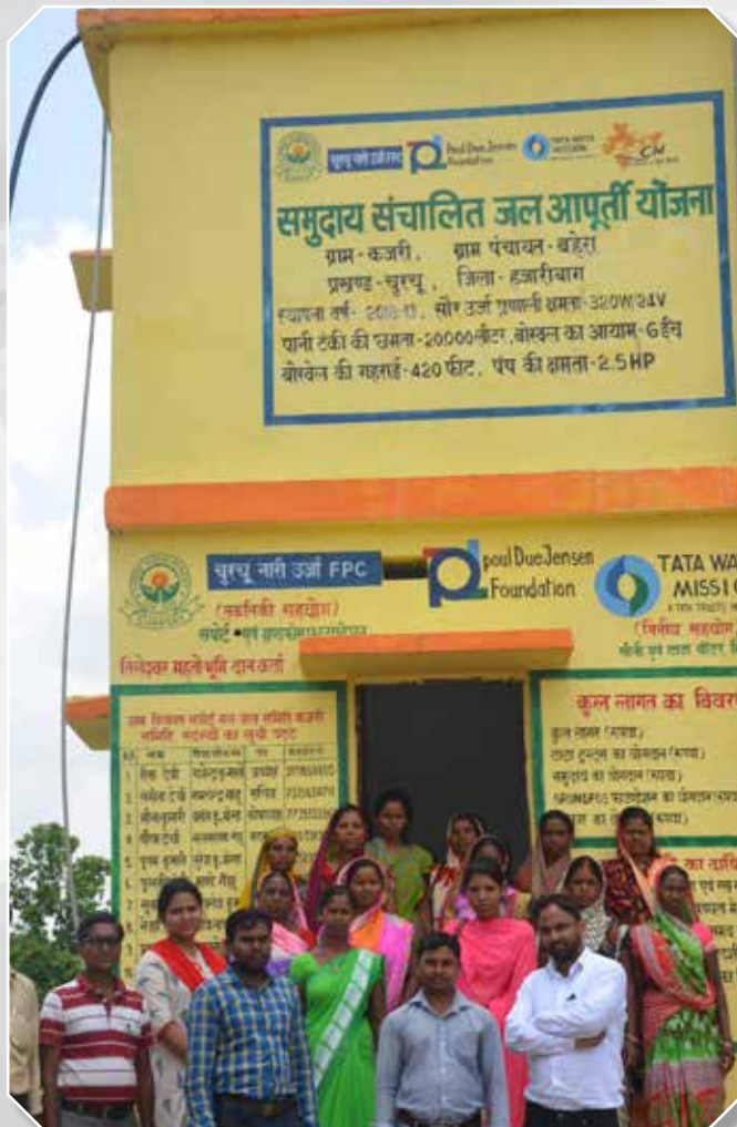
Water Tank at Kajri, Churchu, Hazaribagh
