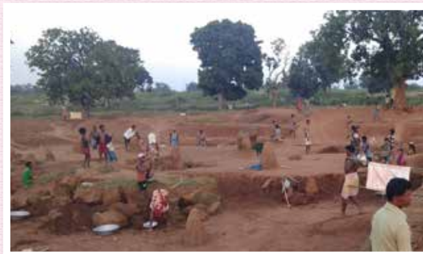
Pond Construction under NABARD-KOH Watershed, Petarwar, Bokaro
